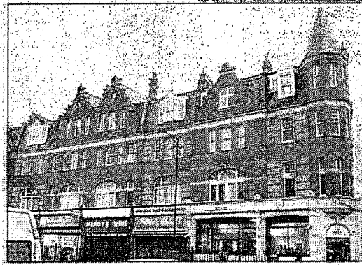
Repairs: Some residents of Streatham Mansions, Streatham Hill, are among those who will receive bills
